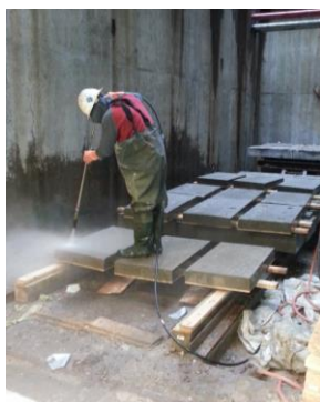
b) high pressure (5500 psi) water wash
