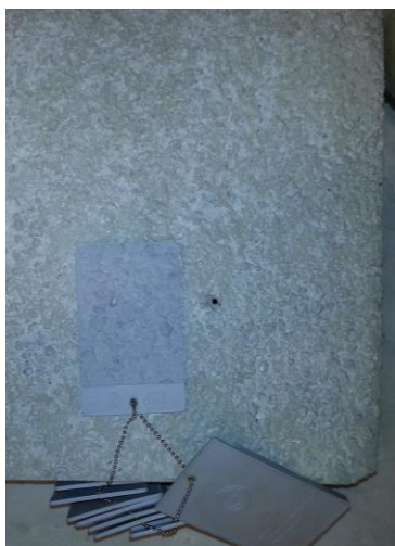
a) surface condition following preparation (CSP8 shown)
