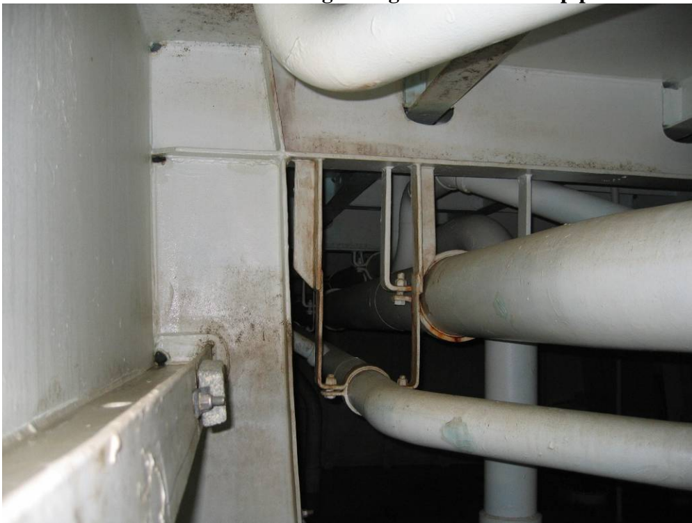
Note the mildew that has formed on various surfaces. This tank appears to stay continually damp. All corrosion noted originates from pipe bracket interiors.
