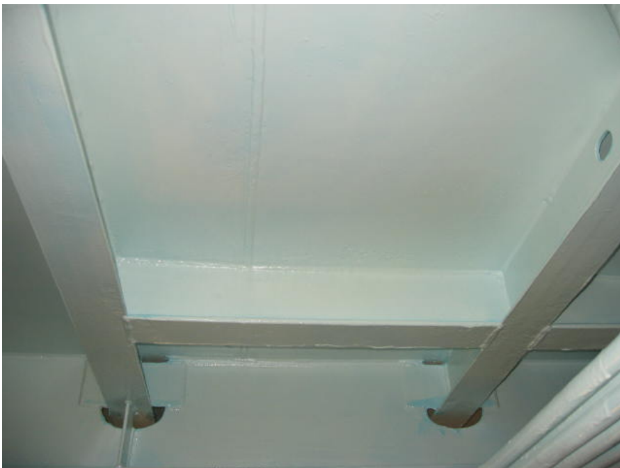
Figure 4 USS OAK HILL (LSD-51) Final Coat Applied 3-121-1-W
