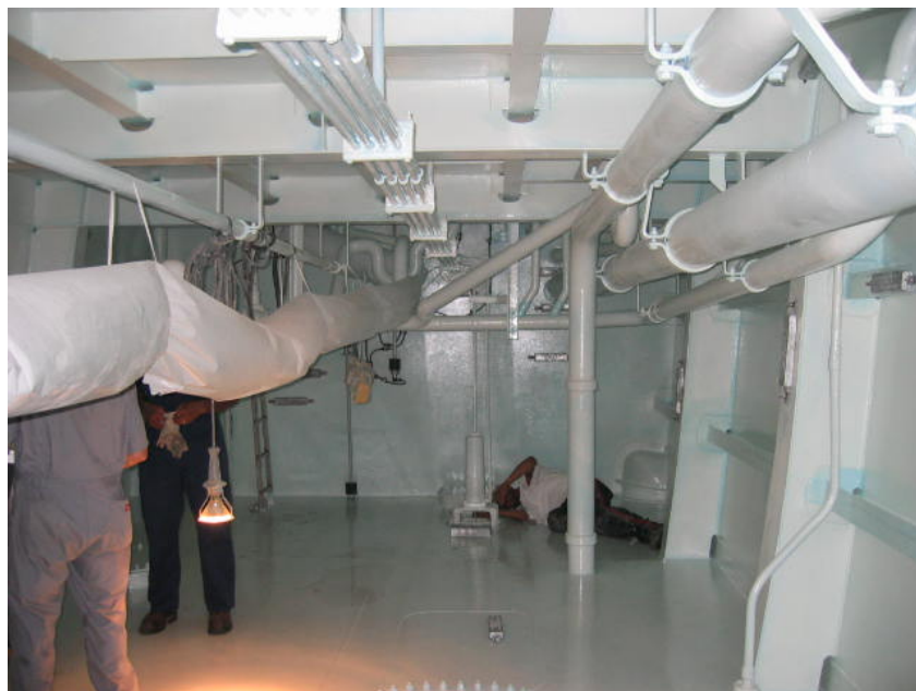
Figure 6 USS OAK HILL (LSD-51) Final Coat Applied 3-121-1-W
