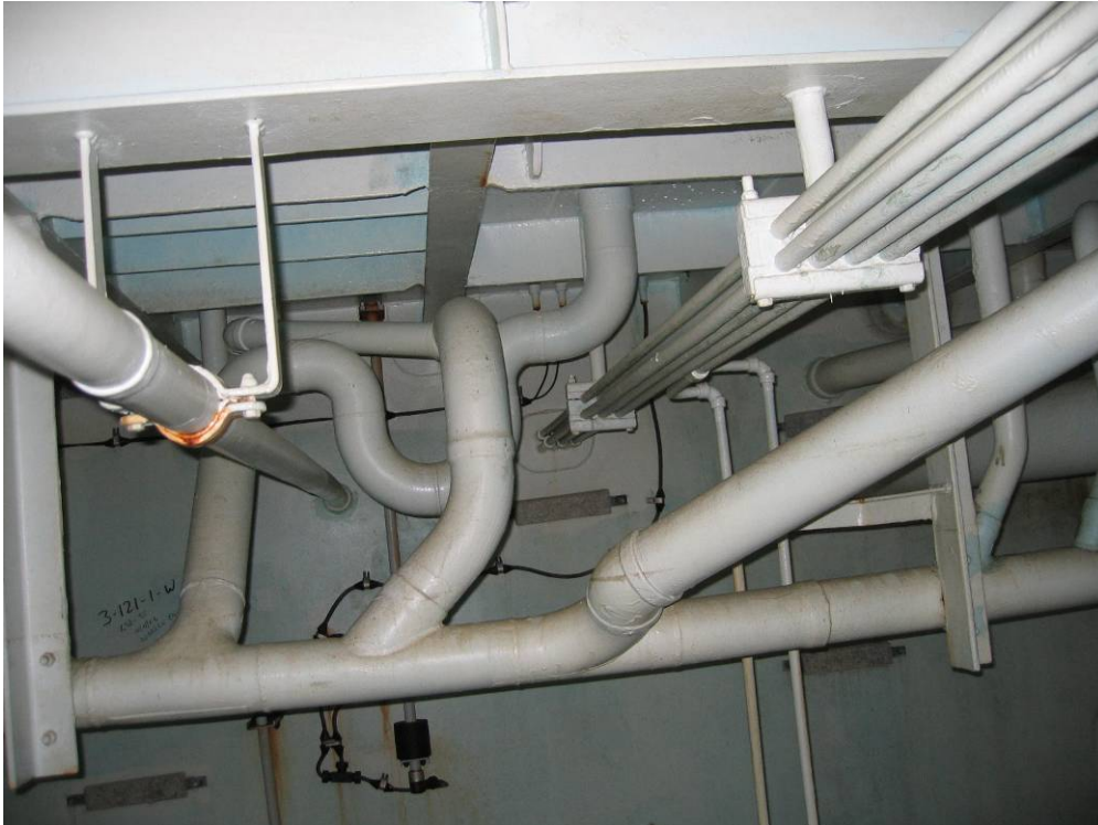
Overhead at Forward end. Corrosion seen on the Forward Bulkhead in way of the Tank Level Indicators (TLI's) originates with uncoated mating surface of the mounting brackets.
