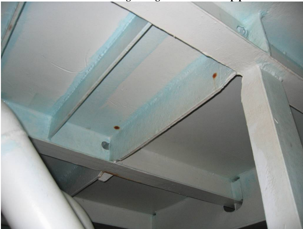
Note the two spots of corrosion. These are deep pits where the coating did not flow into and seal. Note the overall excellent film build on all edges and outside corners.
