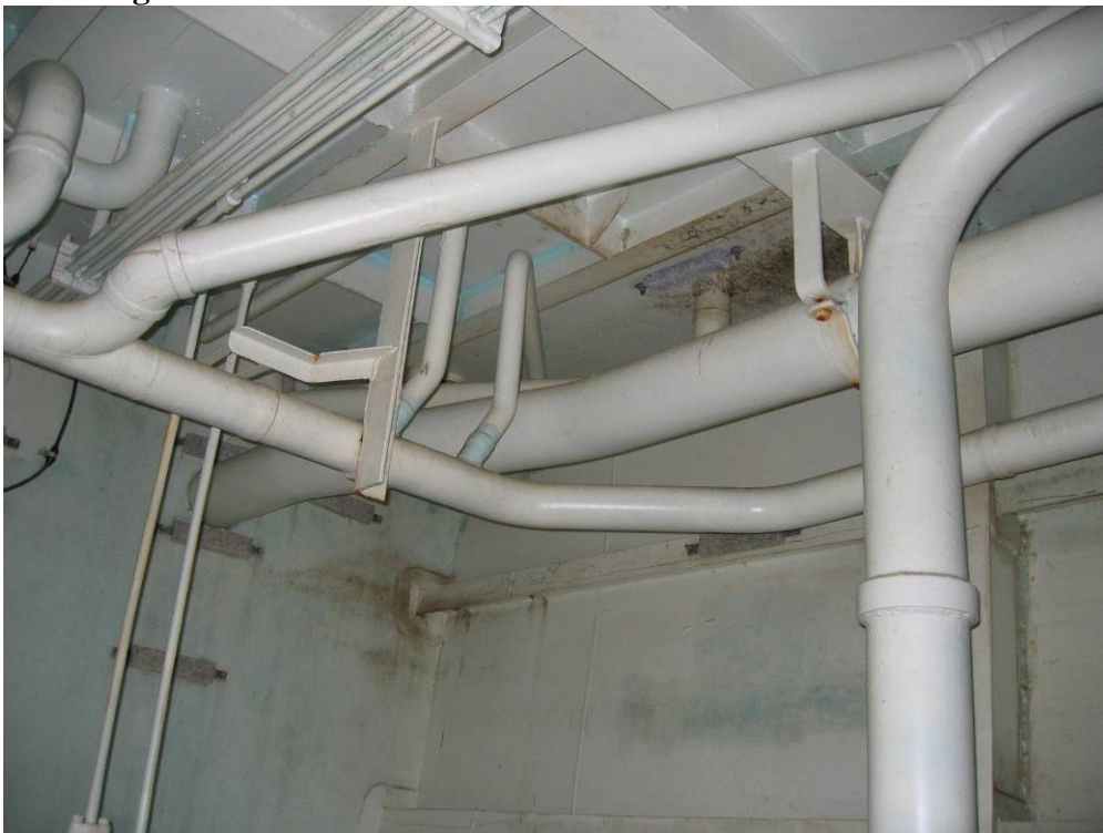
Note the black mildew on various surfaces
