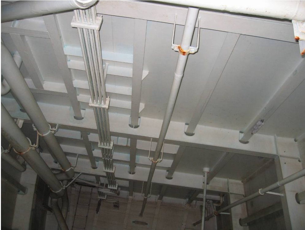
USS Oak Hill LSD-51 SWB Tk 3-121-1-W with Warren Environmental S-301 Rapid Cure coating system applied 15-months earlier. Looking Aft at the Overhead. All corrosion seen is rust stain originating from interior of pipe brackets.
