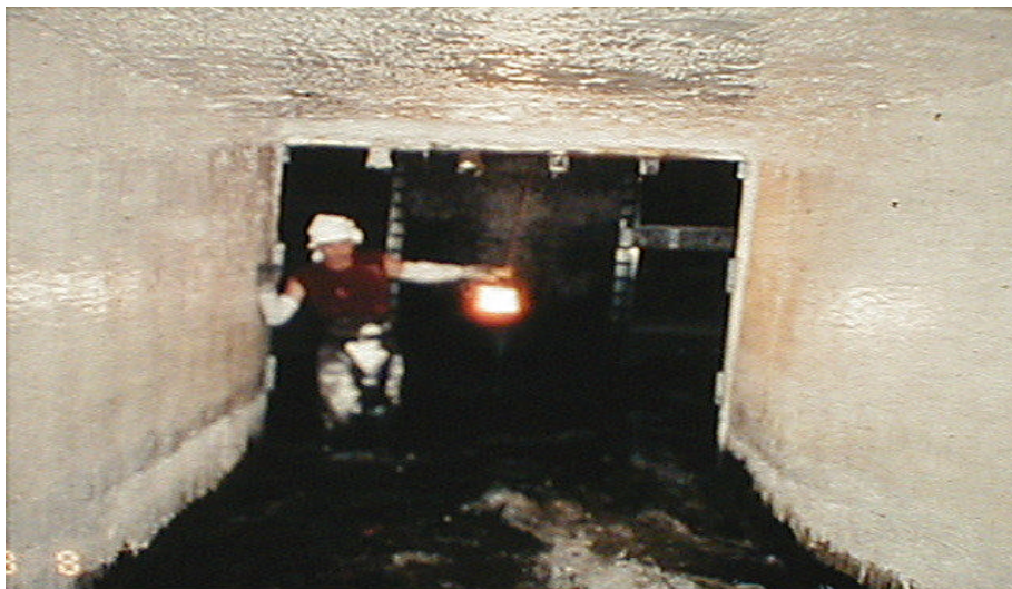
Chlorine washed and power washed prior to two-year inspection – Miami Dade, FL
