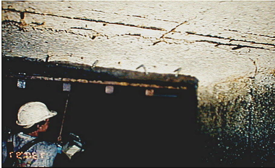
Main pump station collection chamber – Surface prep
