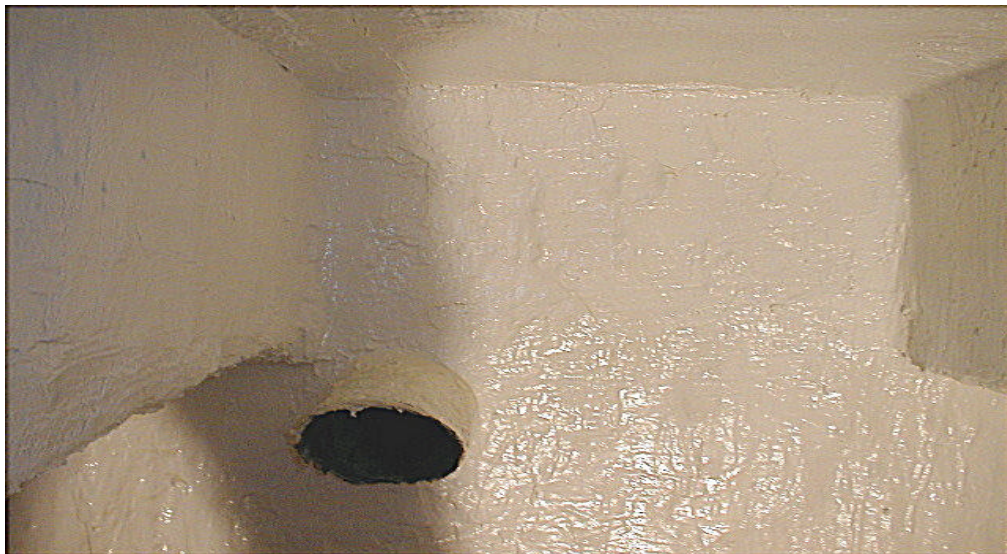
Structurally restored collection tanks with structural epoxy system
