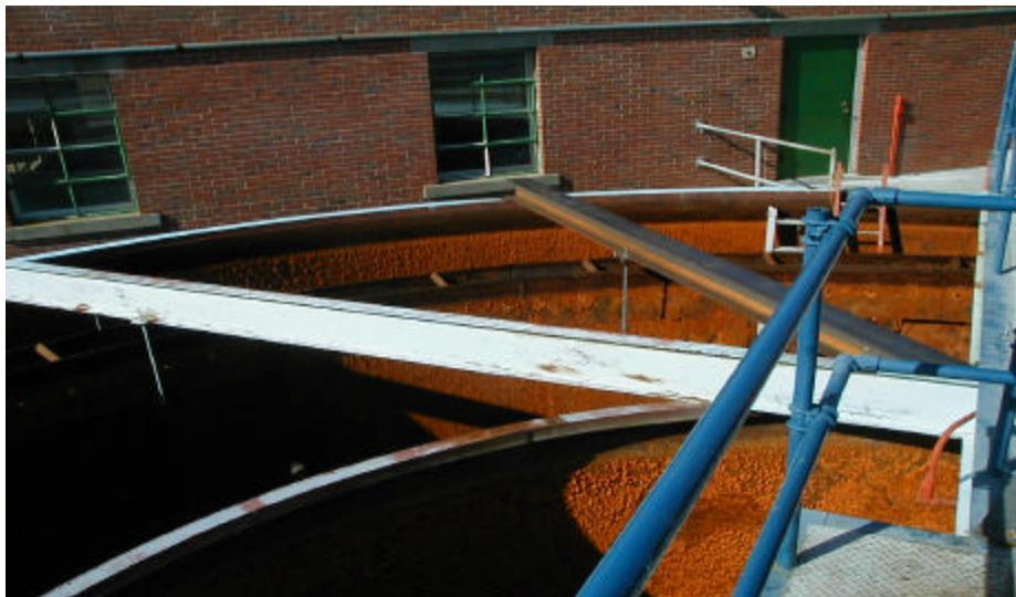
Raw Water Clarifier Tank Prior to Surface Prep
