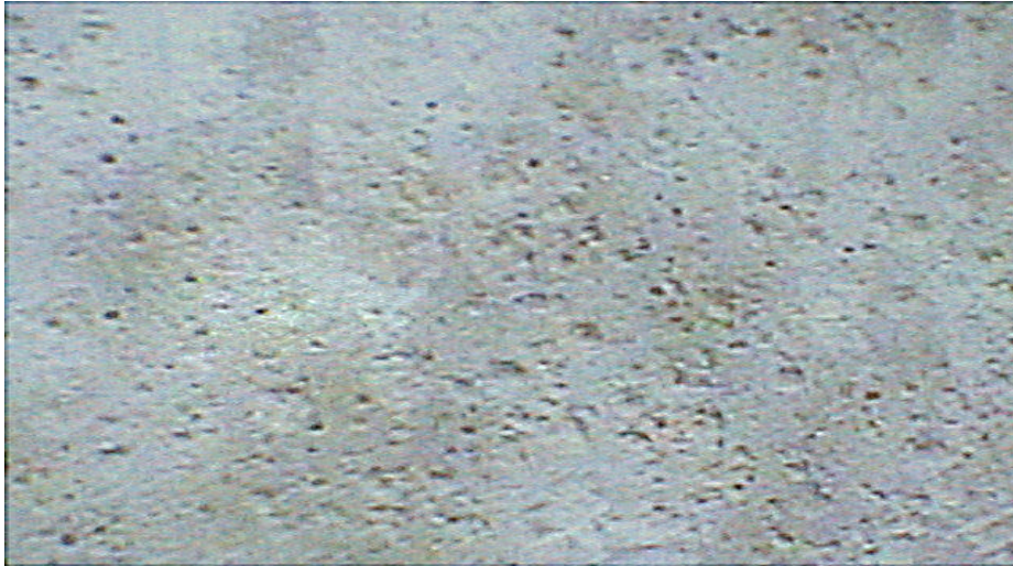
Near white metal blast of clarifier walls
