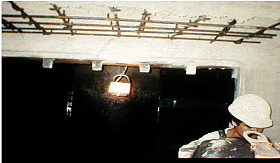
Installation of new rebar where original rebar and concrete substrate had deteriorated back to the earth
