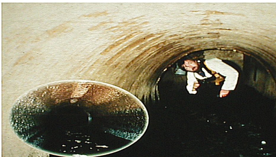
Two-year inspection performed by KTA Tator showing no sign of further corrosion
